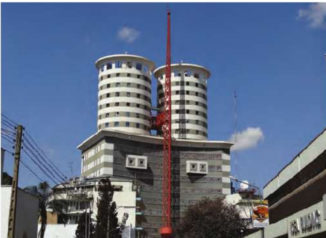
ECL maintains some of the fastest lifts in East Africa, including the 4-mps units at the Nation Centre in Kenya.
